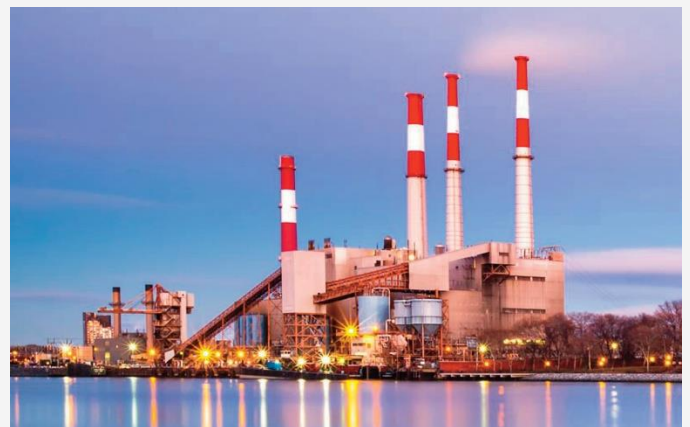
Ravenswood Generating Station. Credit: Rise Light & Power, LLC
